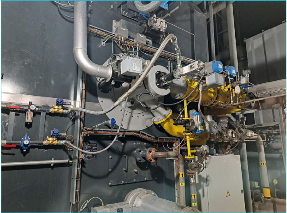
Abb. 4: Installation ELCO RPD 60 GG-EU1 HL an Cannon-Bono OMP10000
